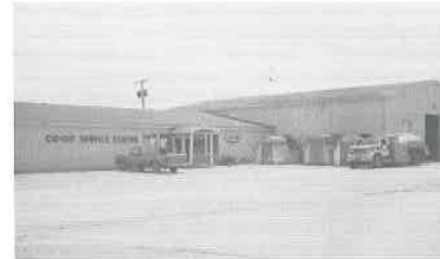
CO-OP Service Centre Complex on the Trans-Canada Highway.
