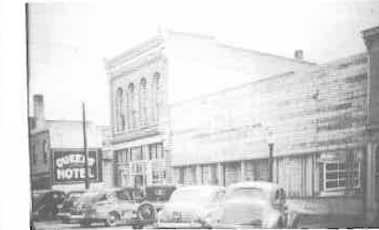
The CO-OP store on main with the new addition to the south under construction.
